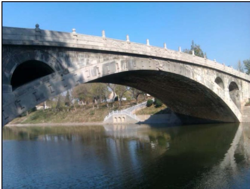
Zhaozhou "Arch" (Anji) Bridge 赵州桥
